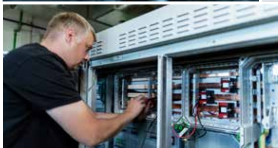
Installing electrotechnical assemblies
